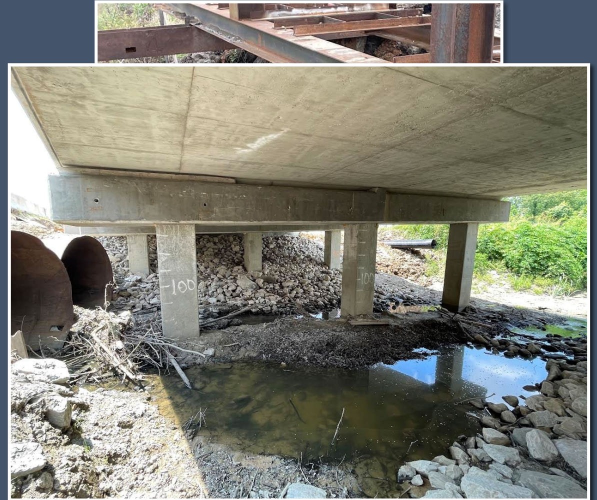
Underneath of Concrete Bridge
