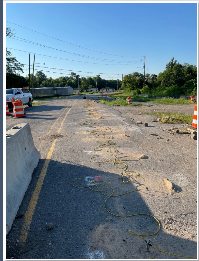
Survey of South Ave (for on bridge)
